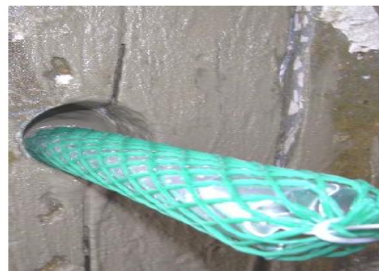
Fig. 5 Anode being placed in grout filled hole [20].
