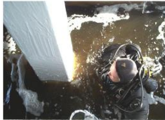
Fig. 2 Fiber reinforced polymer wrap using divers [43]
