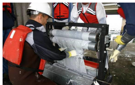
Fig. 3 Mechanically saturation FRP on site [20]
